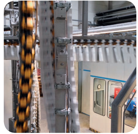
The new post processing system also requires a large amount of compressed air.
