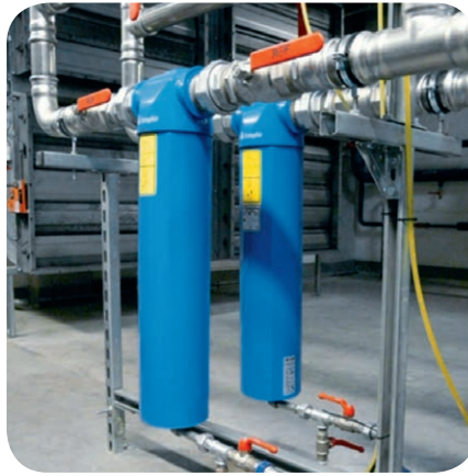
The refrigerant dryer and the upstream and downstream filters were also supplied by CompAir.
